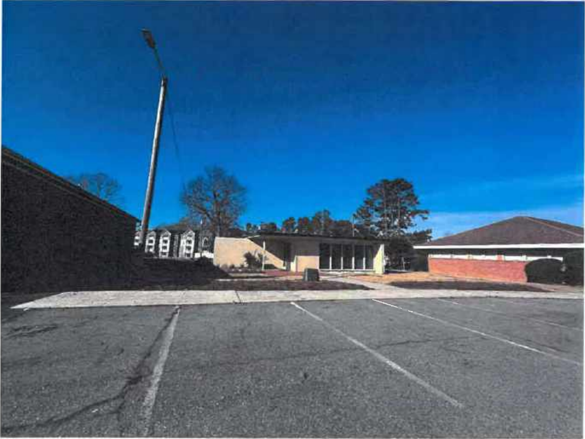
View of the site from Hospital Road
