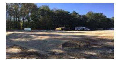
Existing Stone Pad – over 300 tons of compacted process fill material was used in the construction of pad by PW Staff
