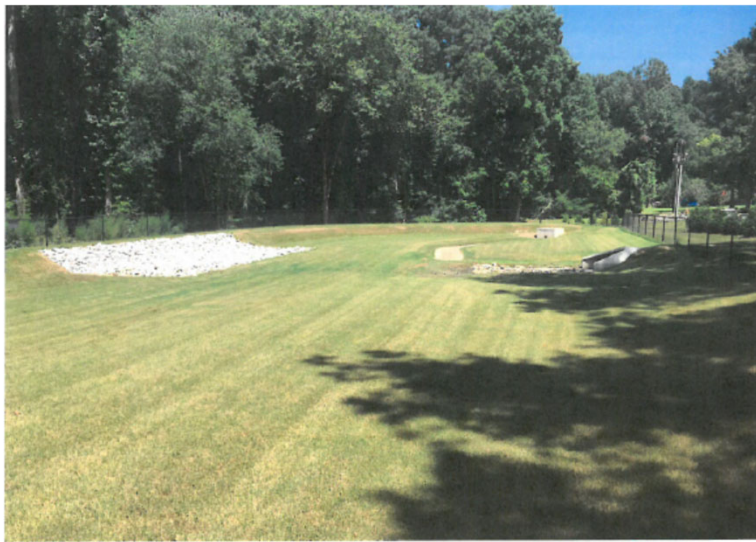
Annual SCM Inspection By Licensed Engineer - Yates Place And Zebulon Community Center
