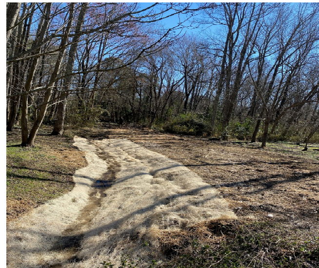
Stormwater Outfall And Ditch Maintenance
