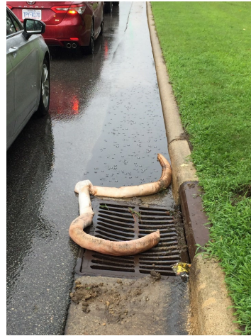
Truck Wreck – Containment Of Fuel Leak
