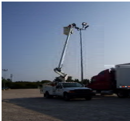
Lighting repairs @ Mudcats
