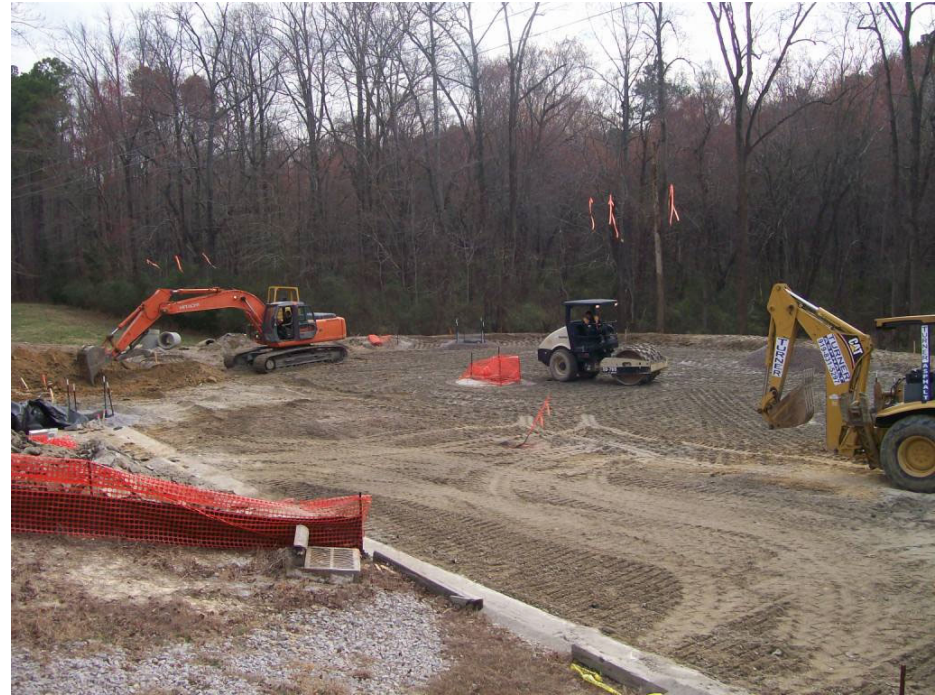
2011 East Barbee Cul-de-sac construction
