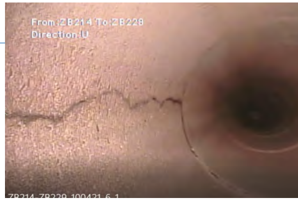
Horizontal cracks
