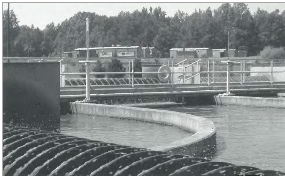
Wastewater treatment plant on NC-39
