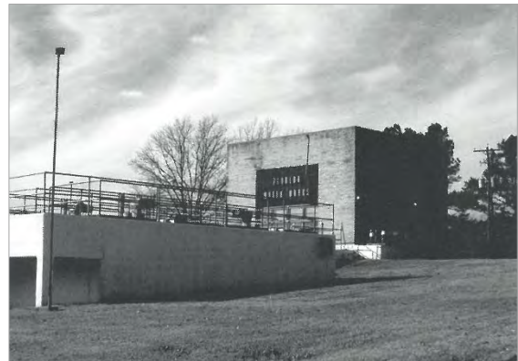
Water plant on the Little River
