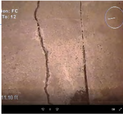
Vertical Cracks
