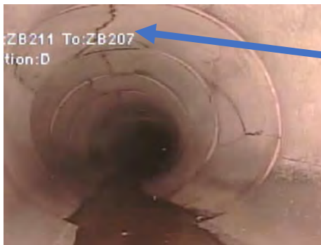
Vertical Cracks
