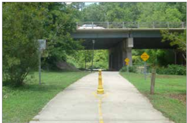
Example of bollard - Chapel Hill, NC
