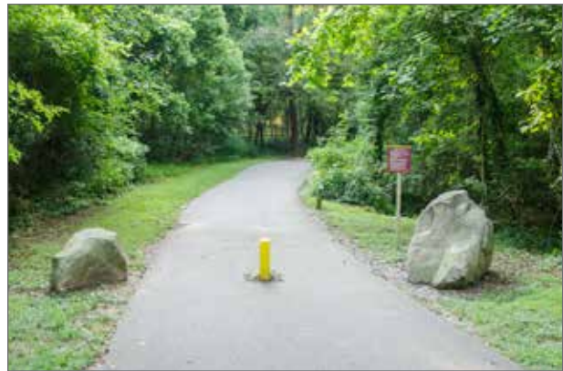
Example of bollard with boulders - Raleigh, NC
