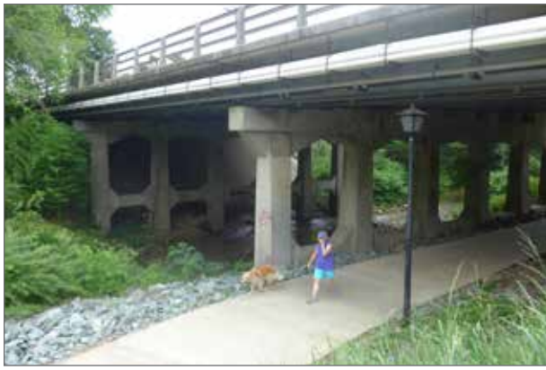
Underpass - Chapel Hill, NC
