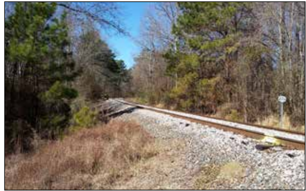
Railroad Corridor behind Five County Stadium
