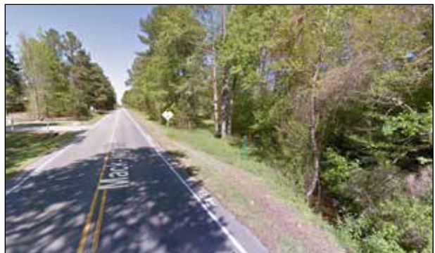
Sewer Crossing at Business 64 (Mack Todd Road) photo courtesy of Google Maps
