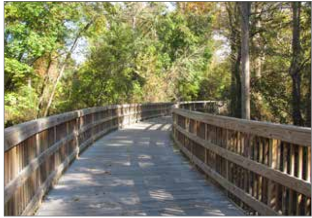
Example of a wooden bridge - Garner, NC
