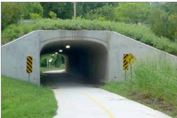
Underpass - Chapel Hill, NC
