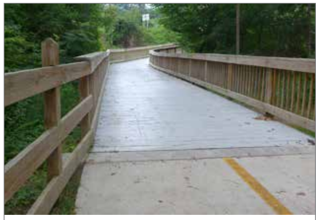
Example of a wood bridge with wood handrails - Chapel Hill, NC
