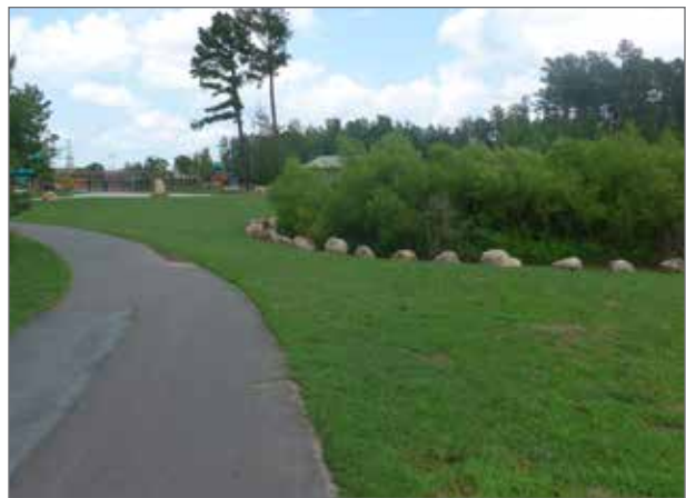
Example of a planted stormwater feature - Chapel Hill, NC
