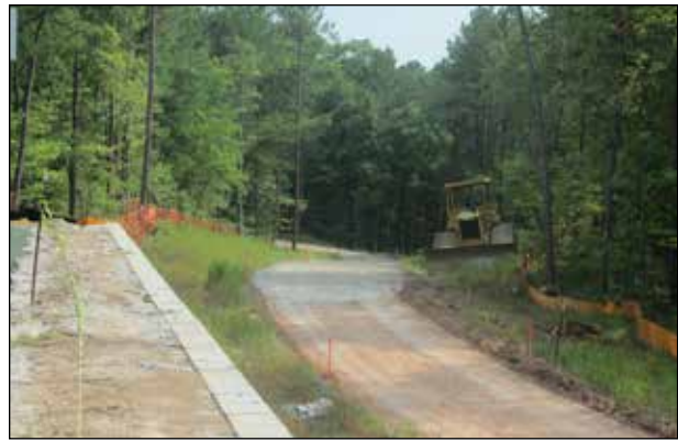
Shiloh Greenway in Morrisville under construction
