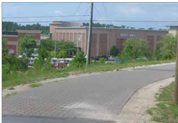
Example of clear site lines - Durham, NC
