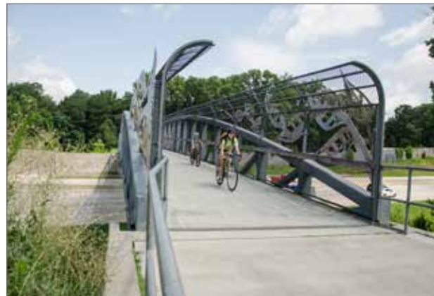
Hinshaw Greenway Bridge over US1/64 - Cary, NC
