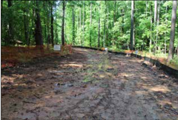
Trail Construction - Raleigh, NC
