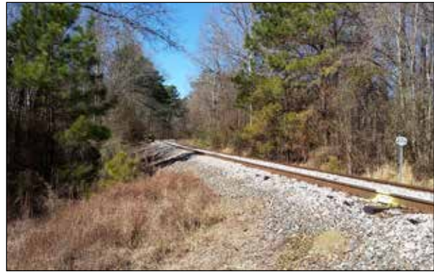
Railroad Corridor behind Five County Stadium
