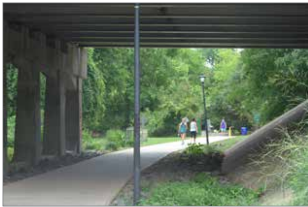
Underpass - Chapel Hill, NC
