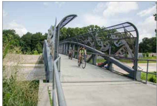
Hinshaw Greenway Bridge over US1/64 - Cary, NC
