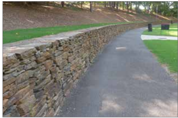
Retaining Wall at the Art Museum - Raleigh, NC
