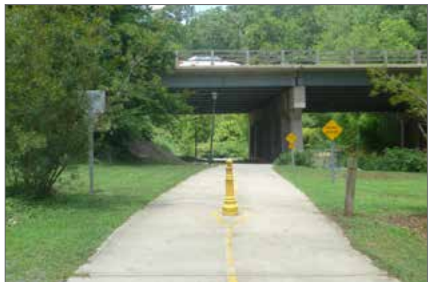
Example of bollard - Chapel Hill, NC
