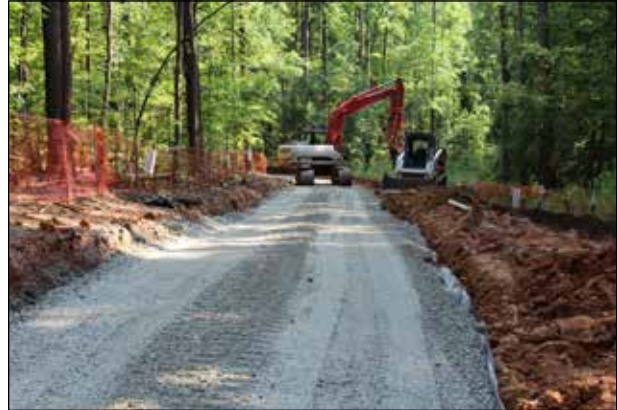
Trail Construction - Raleigh, NC
