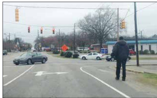
Lack of pedestrian facilities along Gannon Ave. create unsafe conditions.
