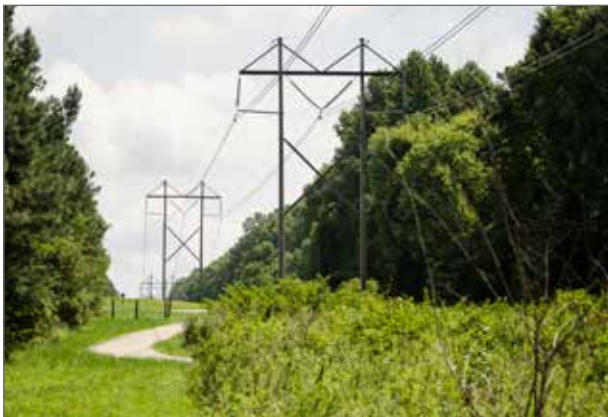
Trail within Power Easement
