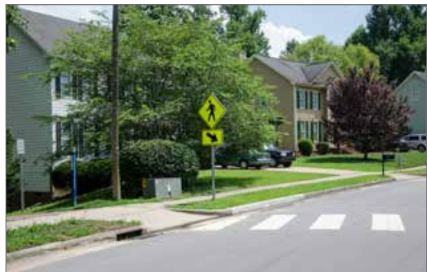
Crosswalk with standard MUTCD signage - Cary, NC
