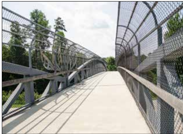
Example of a highway crossing - Cary, NC
