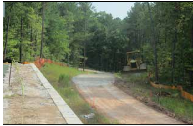
Shiloh Greenway in Morrisville under construction
