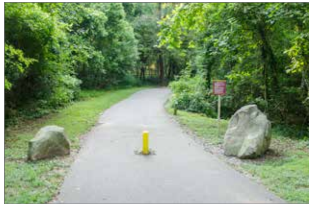
Example of bollard with boulders - Raleigh, NC
