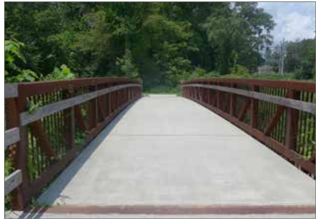
Example of a concrete bridge with corten steel handrails - Chapel Hill, NC
