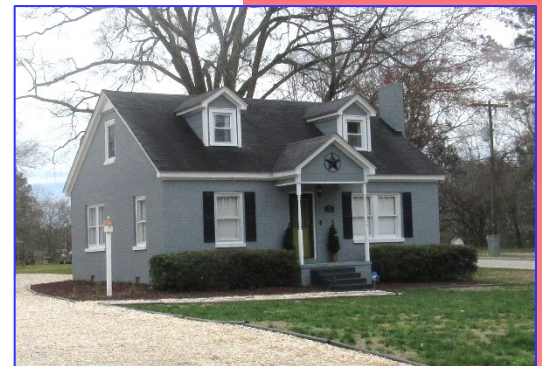
Example of a small footprint home near Downtown, along N. Wakefield Street.
