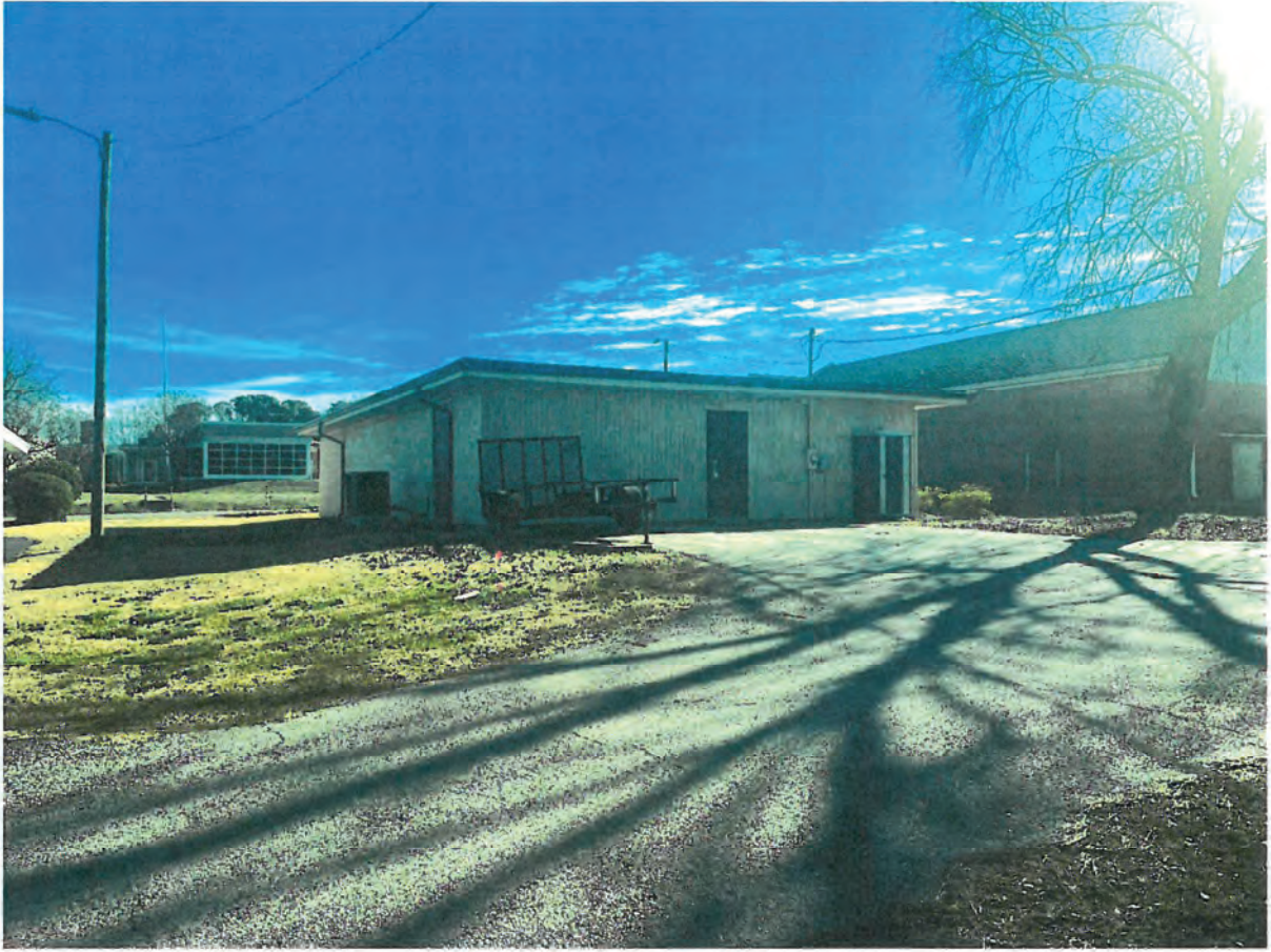
View of the site from Pony Road
