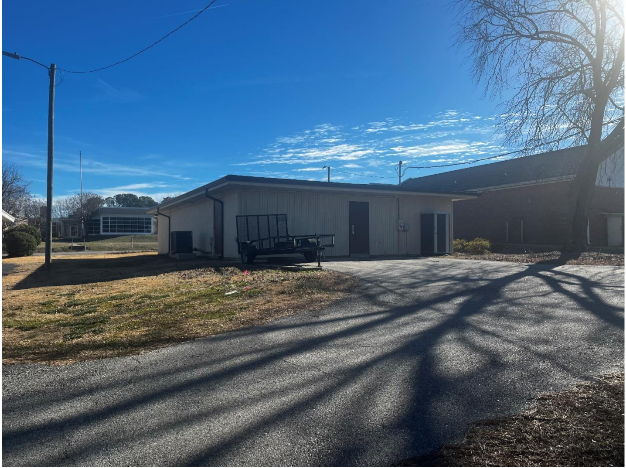
View of the site from Pony Road
