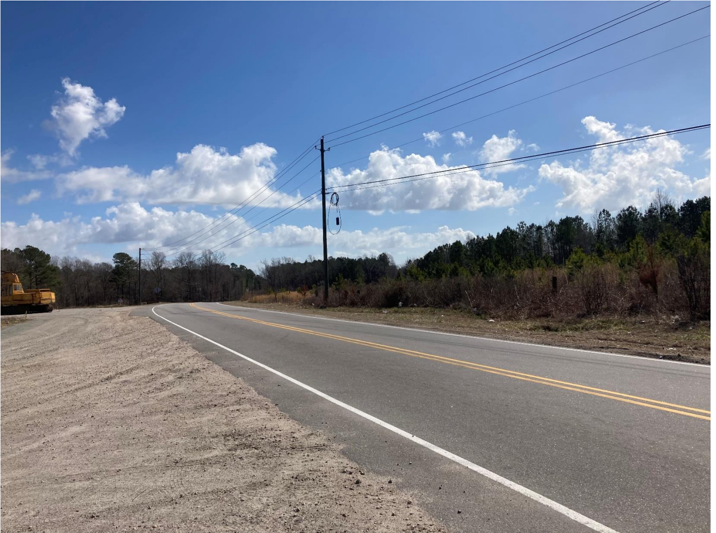
View of property looking down Old US 264 Hwy
