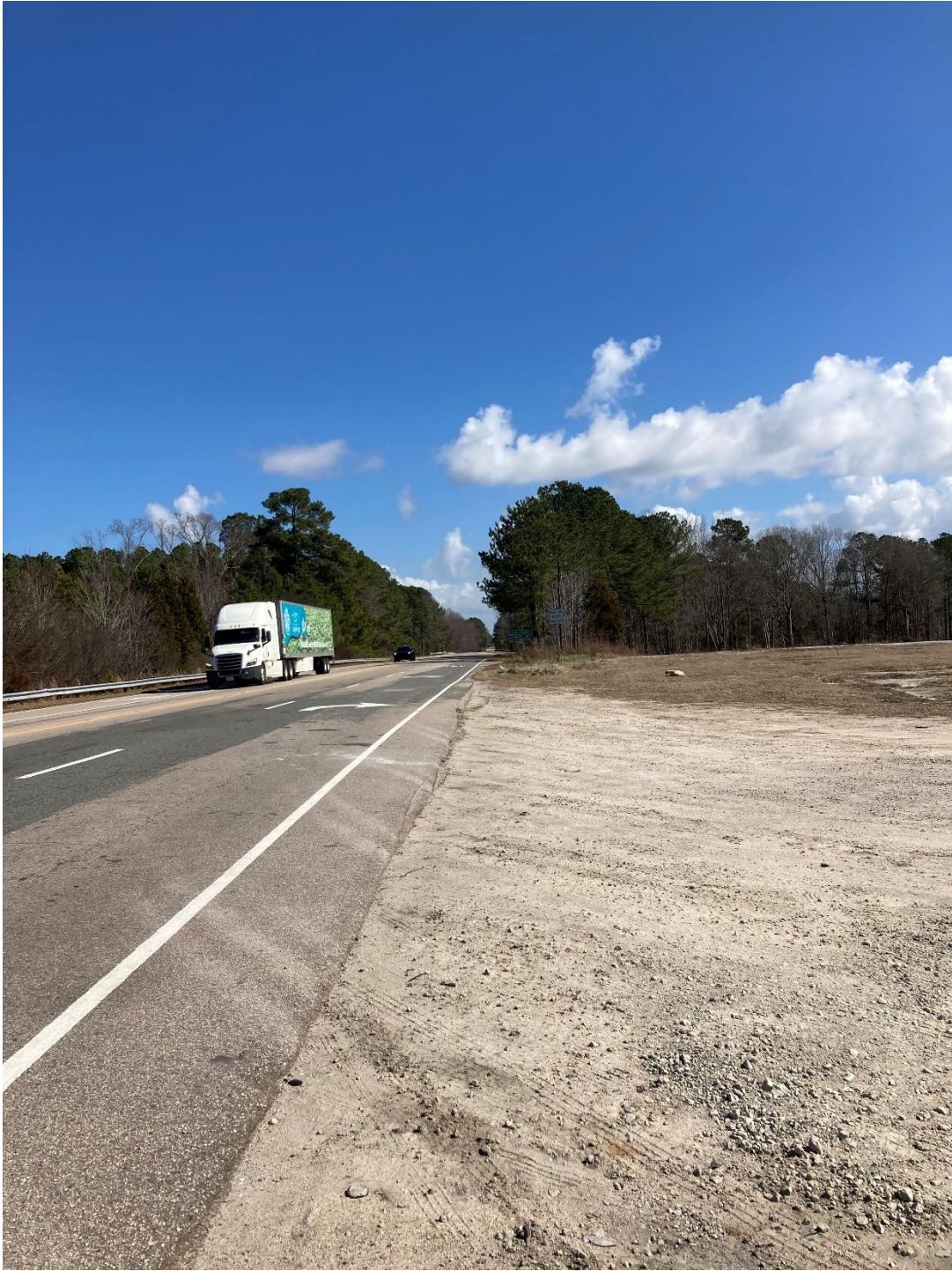
View looking east down E Gannon Ave toward US 264 Hwy
