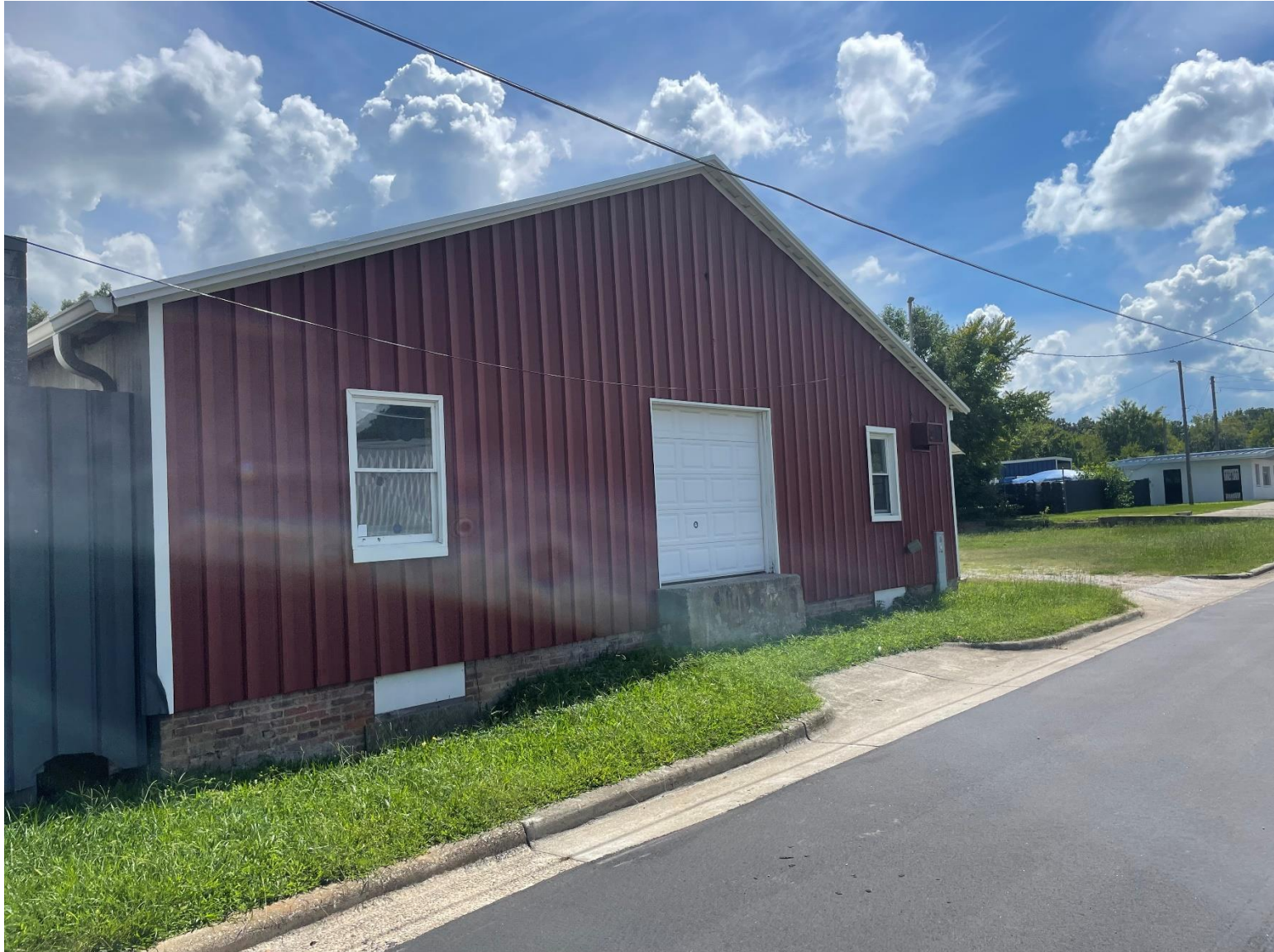
Adjacent building to the right (135 W Vance St)
