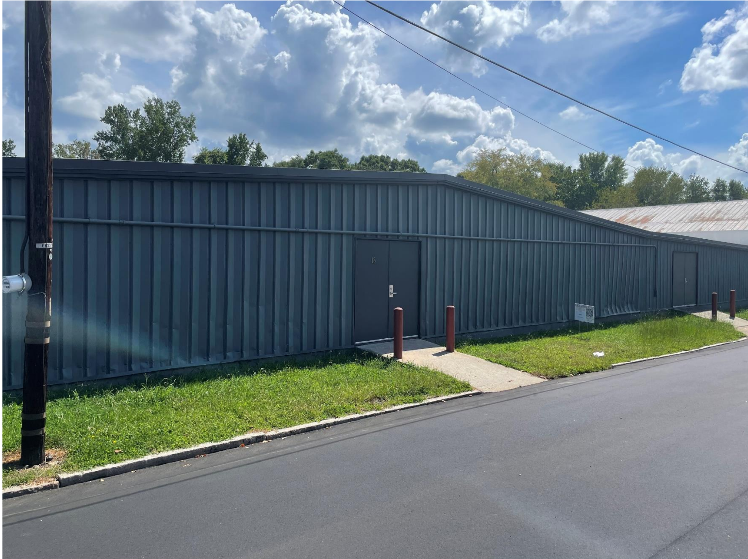
Front of building at 125 W Vance St
