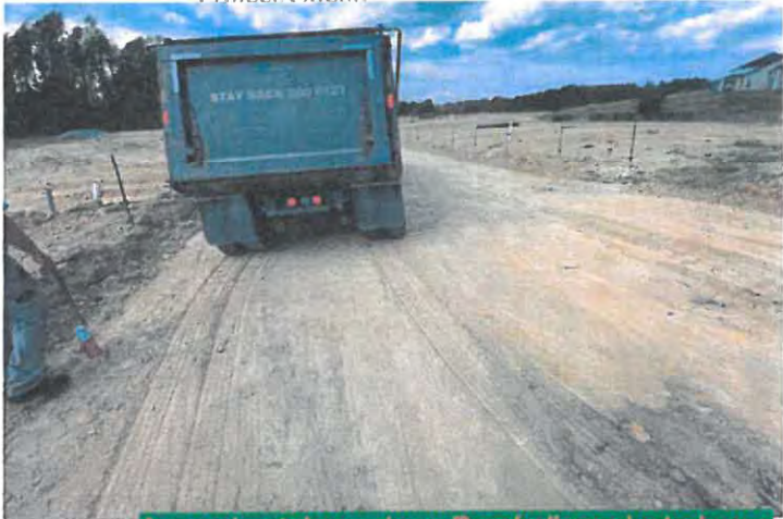
Approximately roadway Proofroll conducted area
