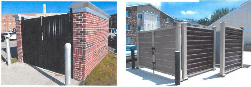
FIGURE 5.3.1.H: COMMERCIAL DUMPSTER ENCLOSURE DESIGN
