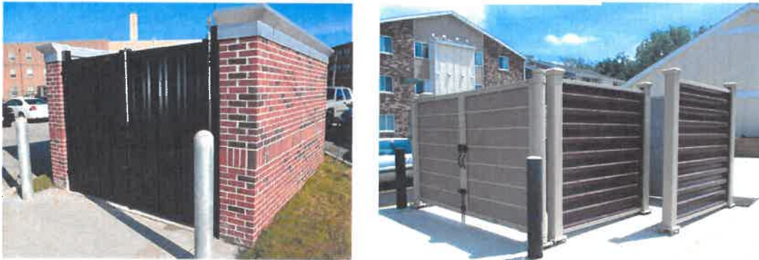
FIGURE 5.3.2.F: MIXED USE DUMPSTER ENCLOSURE DESIGN
