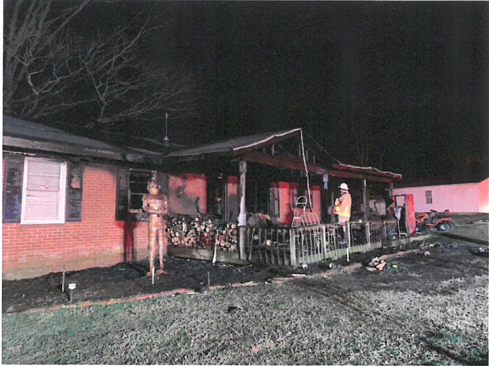
Residential Structure Fire in Carroll Heights subdivision
