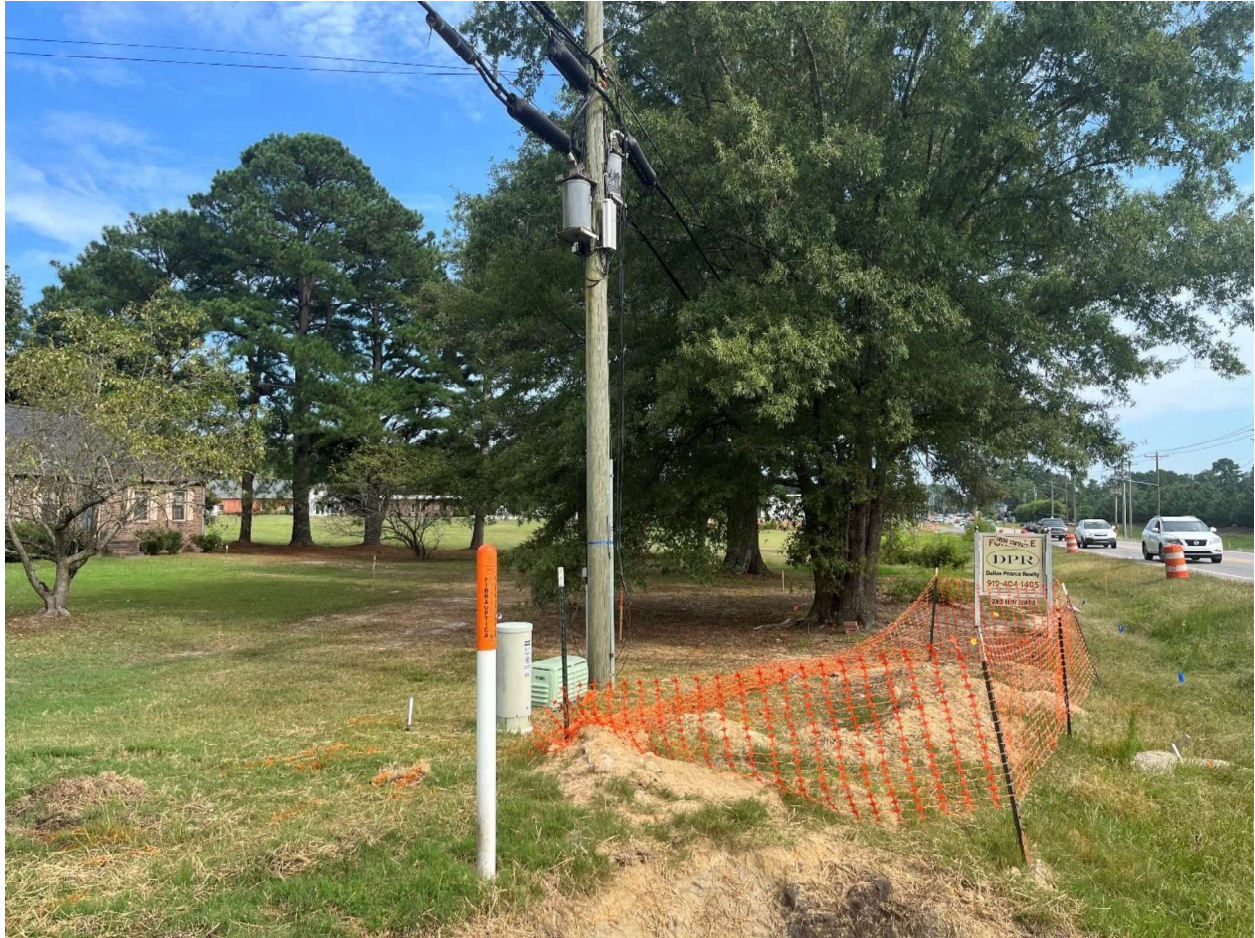
View of the site from the corner of Green Pace Rd and N Arendell Ave looking down Arendell Ave
