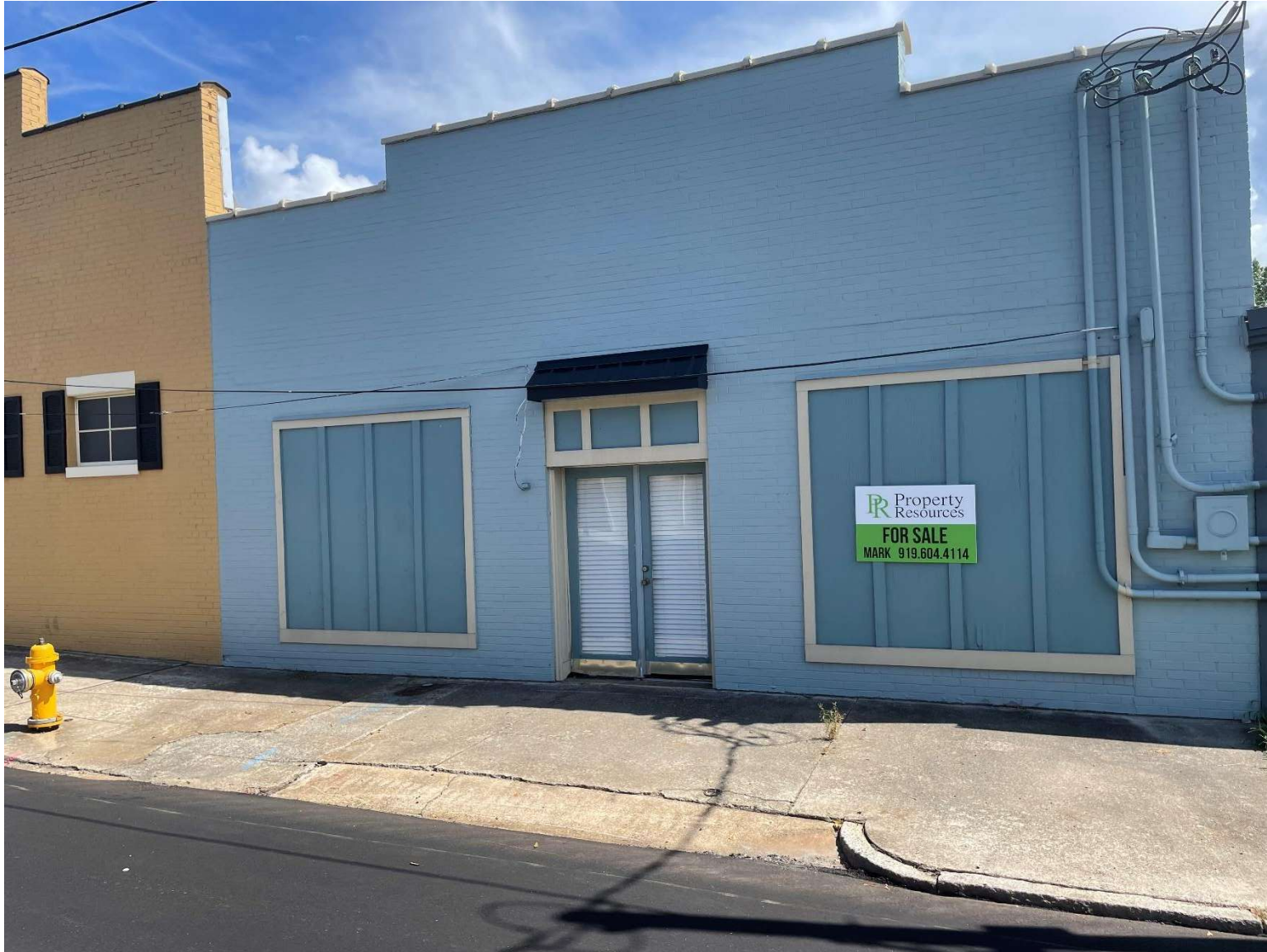
Adjacent building to the left (121 W Vance St)
