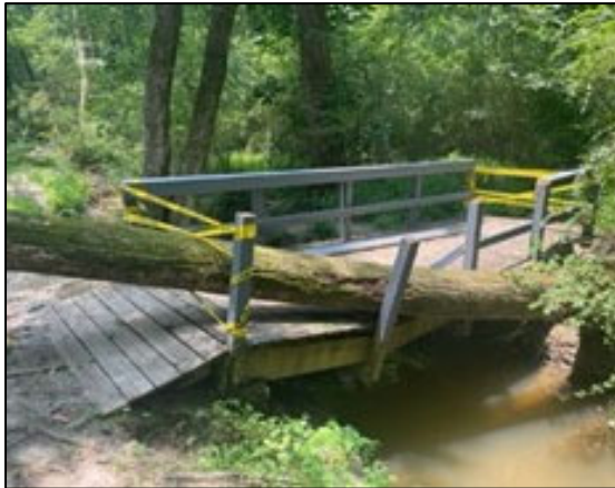
1. Collapsed pedestrian bridge connecting Community Park to Barbee Street.
