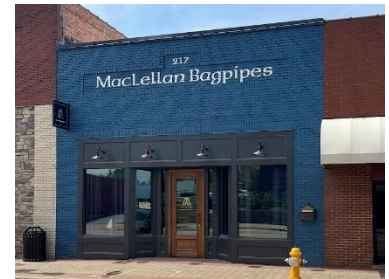
Downtown Building Renovations:
