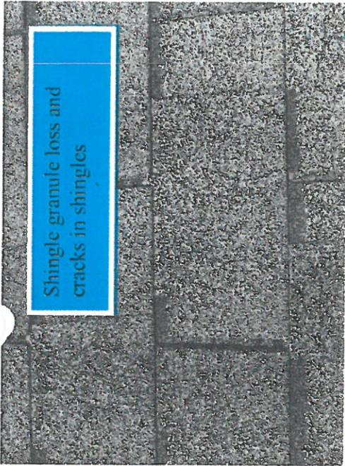
Shingle granule loss and cracks in shingles
