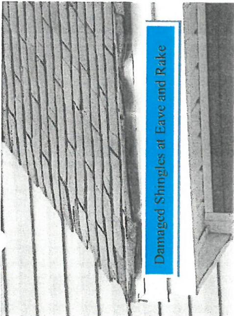
Damaged Shingles at Eave and Rake
