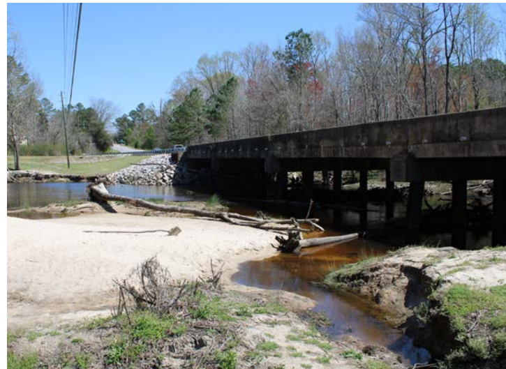
Daylighted Stormwater Channel
