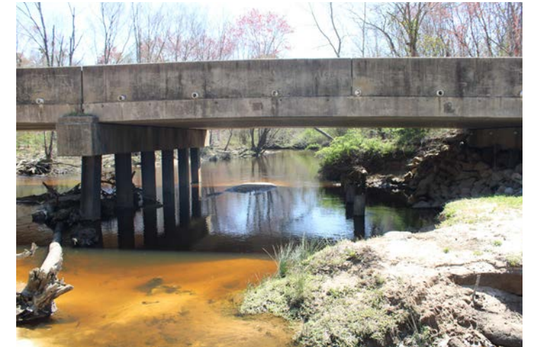
Little River Under the W Gannon Ave/NC 97 Bridge
