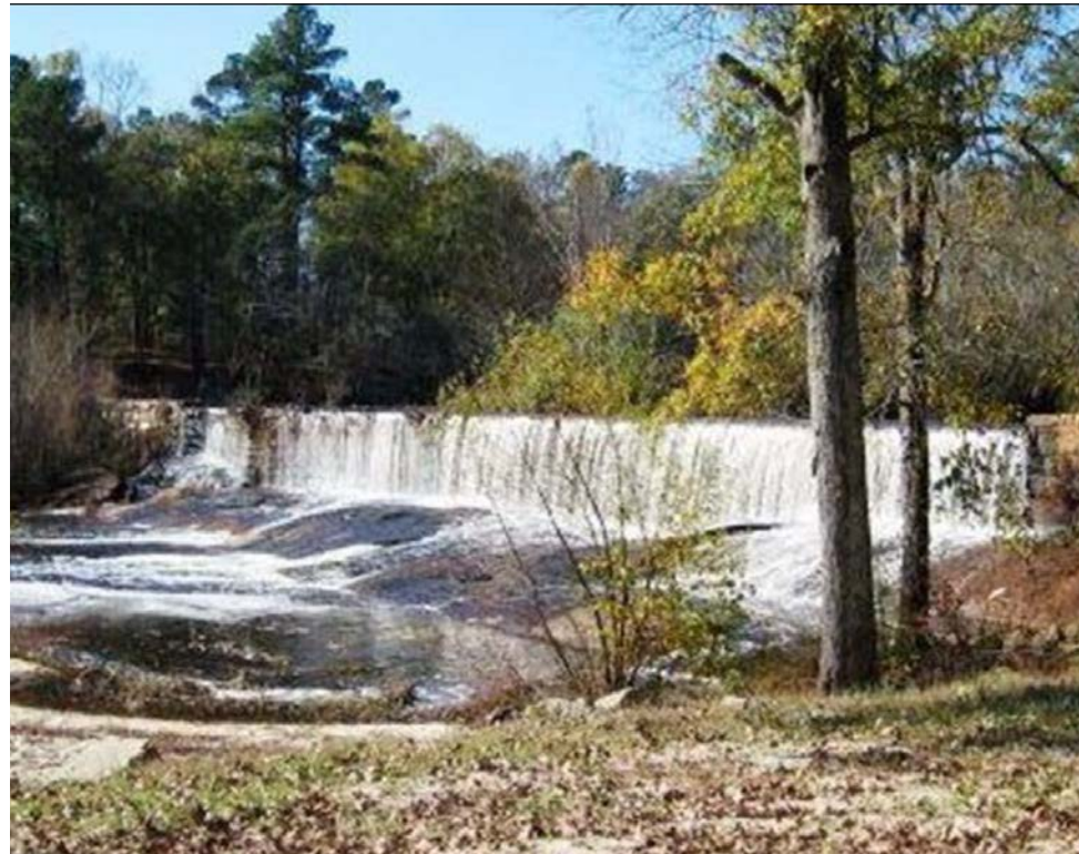
Moore's Mill Dam Before Current Damage
