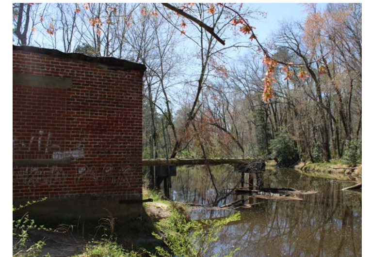
Existing Pump Station
