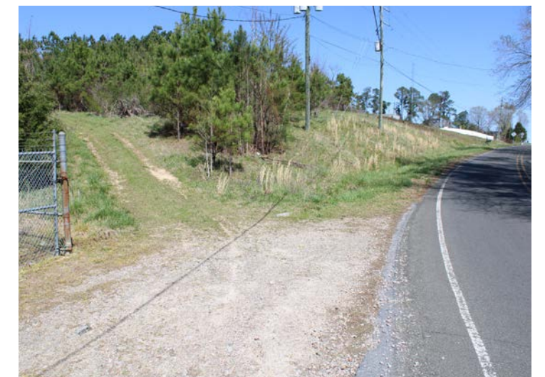
Service Road (unpaved)
