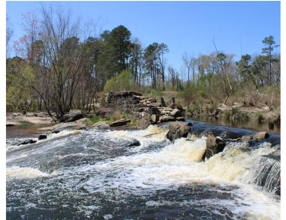
Existing Condition of Moore's Mill Dam
