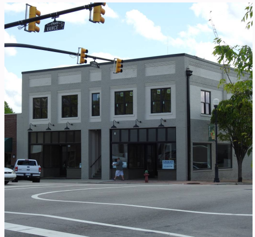
Ashbrook Builders completed a $180,000 renovation at 104 E Vance Street.
